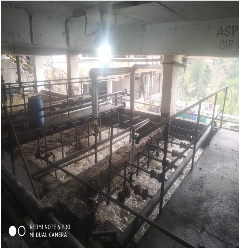
Photo-5: Activated Sludge Process (ASP) Plant 60 KLD
