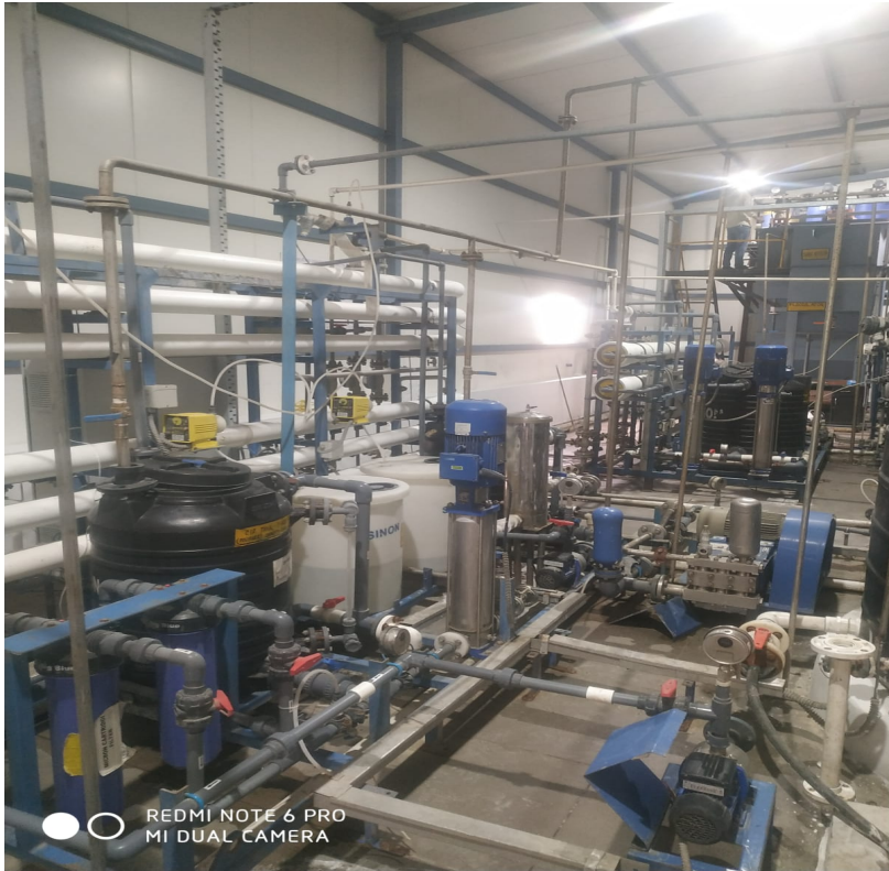
Photo-4: Reverse Osmosis (R.O.) Plant 60 KLD
