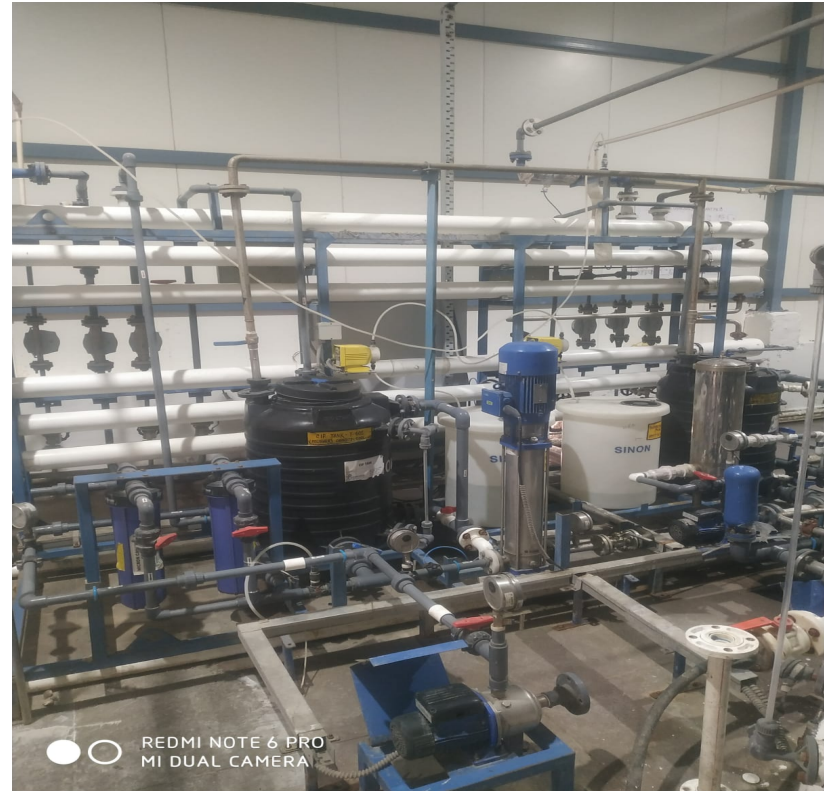
Photo-4: Reverse Osmosis (R.O.) Plant 60 KLD
